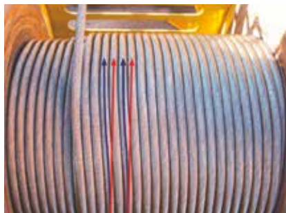
Figure 60 - Proper spooling (no gap between the wraps)
