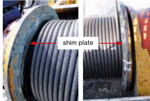
Figure 52 - shim-plate on drum
