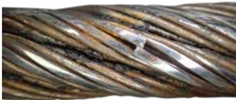
Figure 74 - Crown wire breaks
